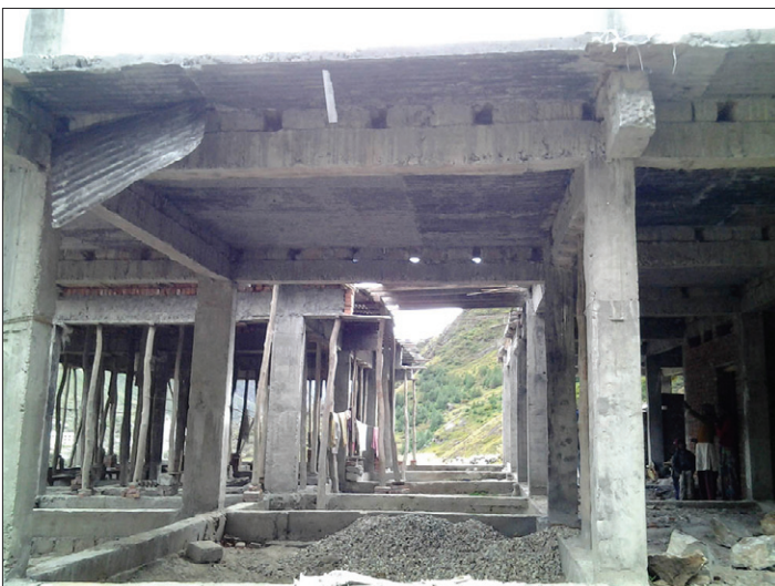
Cement slab ceilings for meditation hall on the left, and apartments and their porticos on the right.
